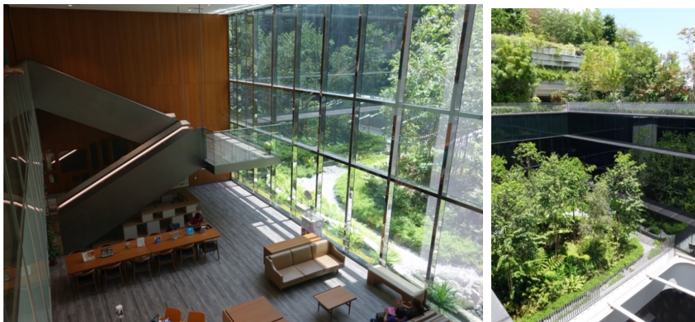
Left: The 4 th floor garden seen from the health care centre. Right: The 4 th floor garden. 3D landscaping and stacked amenities create a vibrant community life in this mix use housing block. Photo: © Françoise Labbe.
