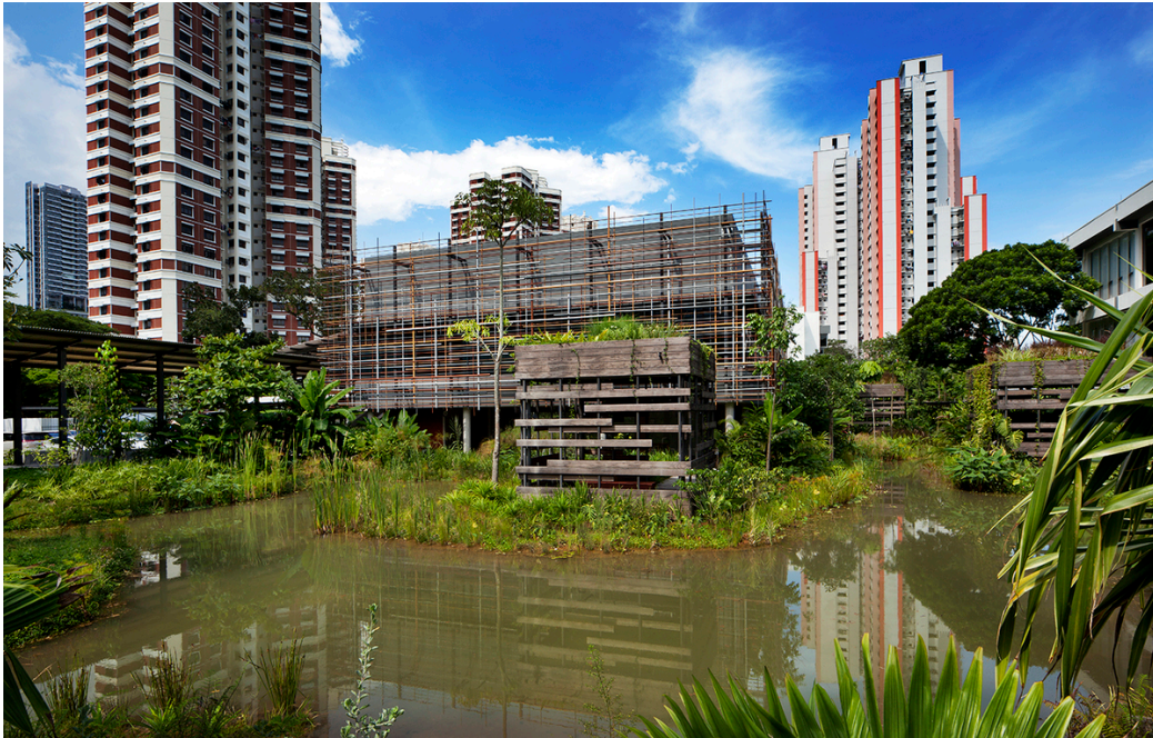
Enabling Village in Singapore, WOHA Architects. Nest Block & Garden Cabana. Photo © Patrick Bingham-Hall.
