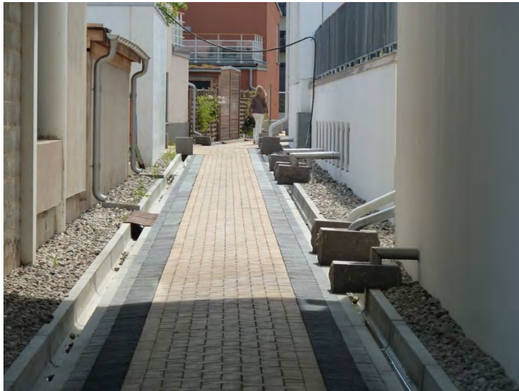
The surface stormwater drainage system at Bo01 features runnels that are less than 25 wide and 35 cm deep. The grating and bridging give access, security, and detailing. The layering of adjacent paving and drainage materials are analogous to patterns in Japanese Zen gardens, such as Ryoanji. Photo: ©Françoise Labbé.
