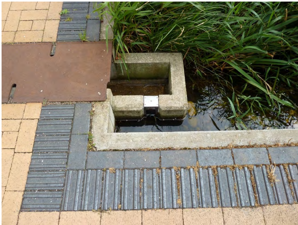
Green and water in Malmö. The infrastructure is revealed rather than concealed from the residents. The granite blocks and edging avoid accidents by heightening visibility. Photo: ©Françoise Labbé.
