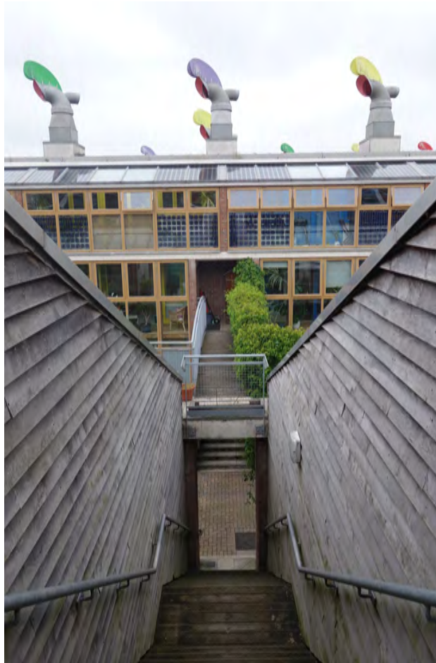
Renewable energy architectural integration in BedZED. Photo: ©Françoise Labbé.
