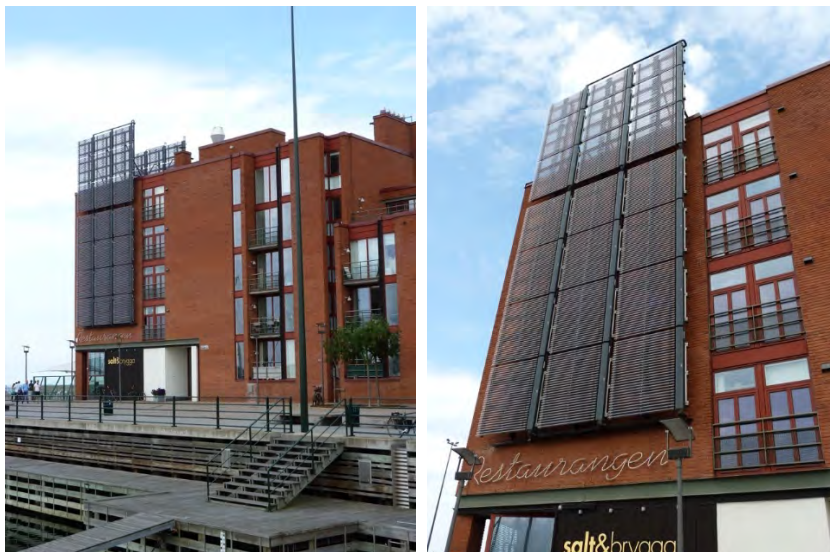
The Tegelborgen building by architect Månsson Dahlbäck features evacuated-tube solar collectors. Photos: ©Françoise Labbé.
