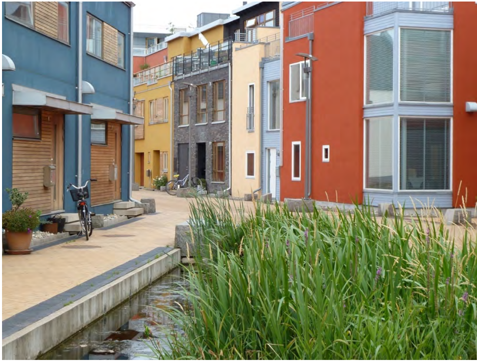
This fresh water marsh within a mixed-use courtyard is an effective stormwater treatment system. The vegetation and presence of water create a contrast with the large paved areas near the Öresund. Photo: ©Françoise Labbé.
