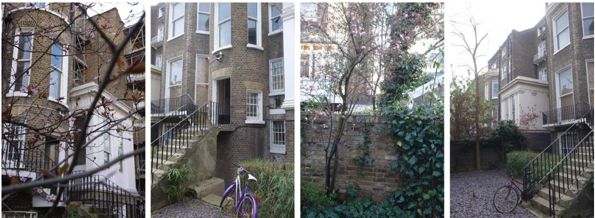
Top: Progression from the house front entrance to its back. Photos: © Françoise Labbé. Bottom: Back of houses in Pembridge Square. Photos: © Françoise Labbé.
