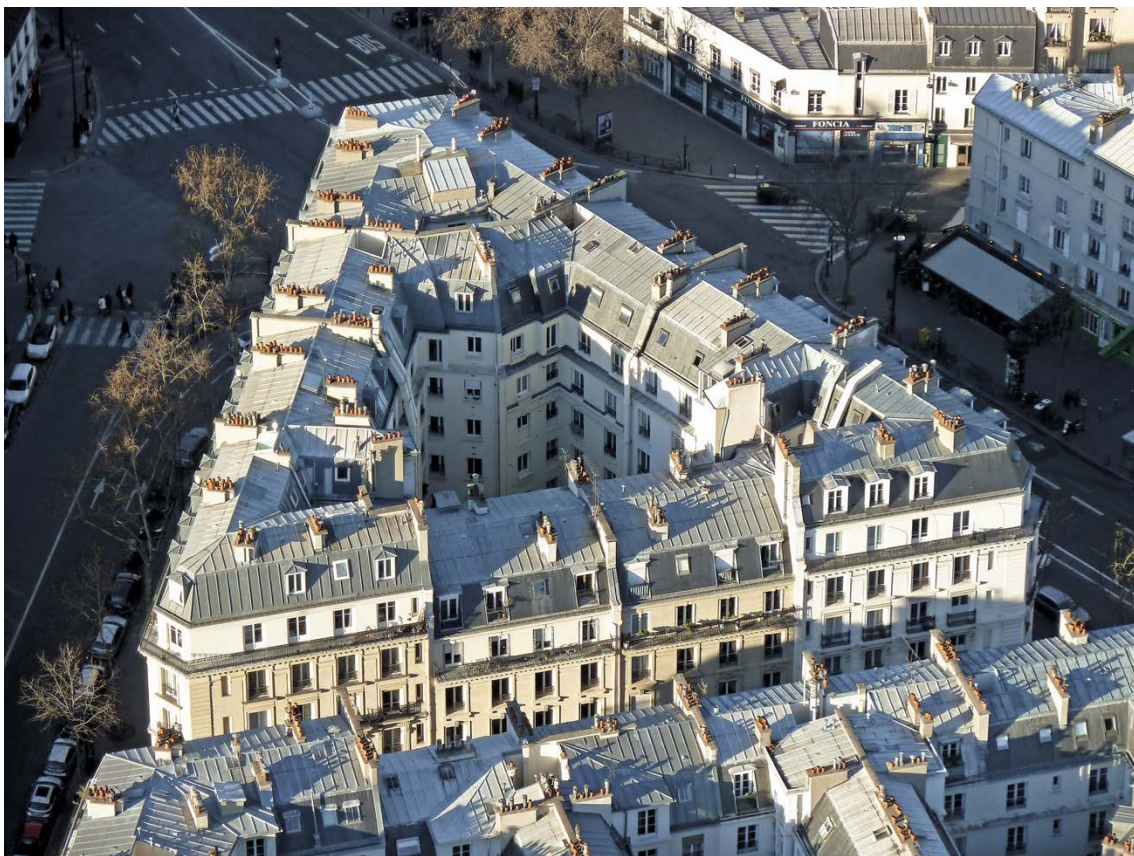
Courtyard perimeter block in Paris. Photo: © Françoise Labbé.
