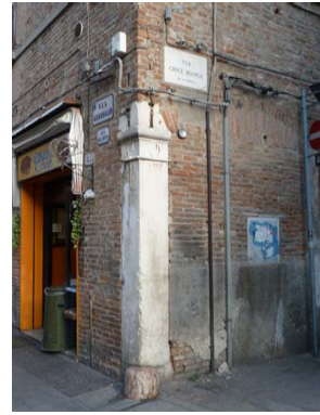
Ferrara. The reinforcement of block corners by white marble pilasters. Photos: © Françoise Labbé.
