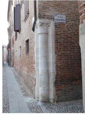
Ferrara. The reinforcement of block corners by white marble pilasters. Photos: © Françoise Labbé.
