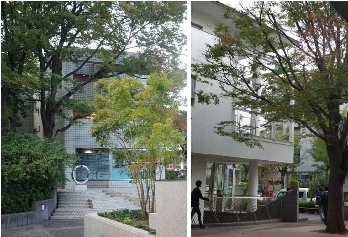
Continuity and evolution over a quarter century. Hillside Terrace. Fumihiko Maki, Architect. Photos: © Françoise Labbe.
